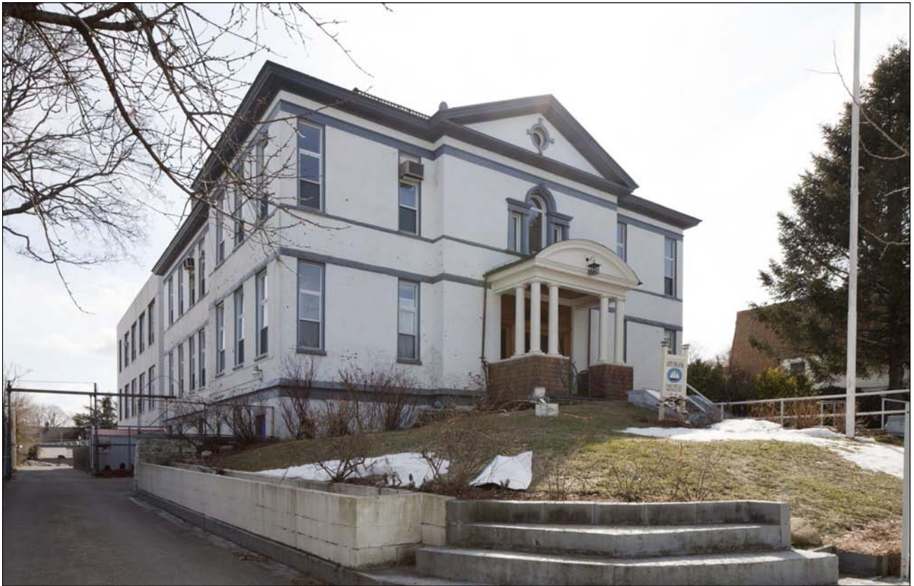
Public School 102 (later Public School 17 — The City Island School), 190 Fordham Street, the Bronx
